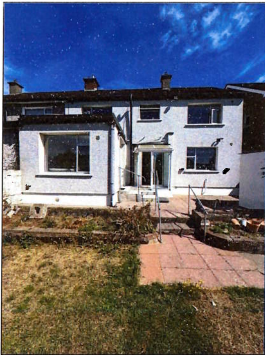
Figure 1 Rear Elevation 7 Woodlands Drive
