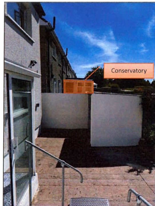
Figure 2 View towards 8 Woodlands Drive
